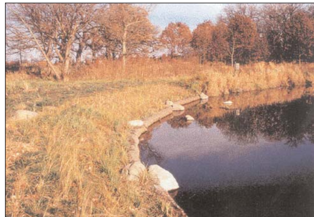
Restoration of a creek meander with adjacent native landscape and public access.
