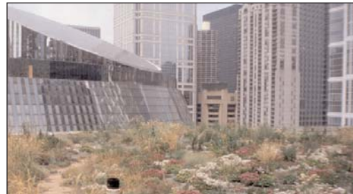
Chicago City Hall green roof insulates the building, provides wildlife habitat, and reduces roof runoff.
