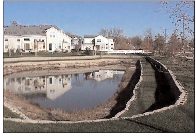
Reliance on conventional detention as a sole stormwater management technique leads to unaesthetic conditions and decreases quality of life.
