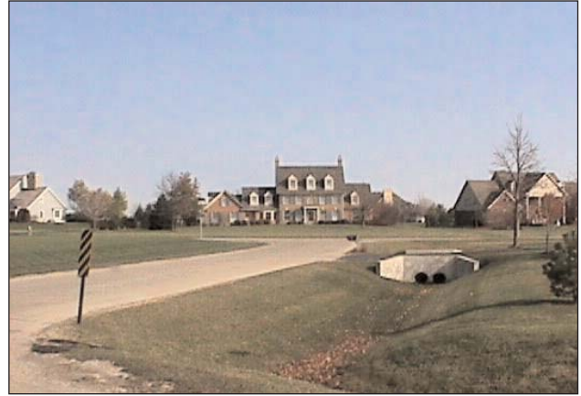
Turf grass stormwater drainage systems often lead to dead grass and bare ground due to wet conditions and subsequent erosion.
