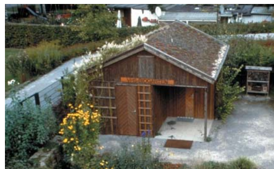
greenroof can be applied on various roofs and scales (Germany)
