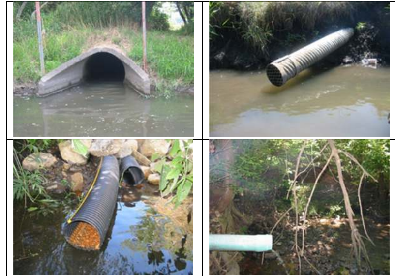
Figure 2-34. Examples of a few of the types of pipes observed discharging to Blackberry Creek during a 2002 stream assessment.
