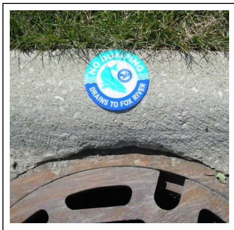
Figure 6-5. Example of a storm drain medallion glued to a curb next to a storm drain inlet.
