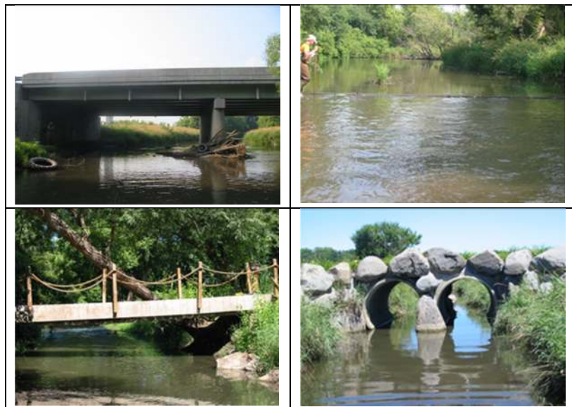
Figure 2-32. Examples of a few of the types of hydraulic structures observed crossing Blackberry Creek during a 2002 stream assessment.
