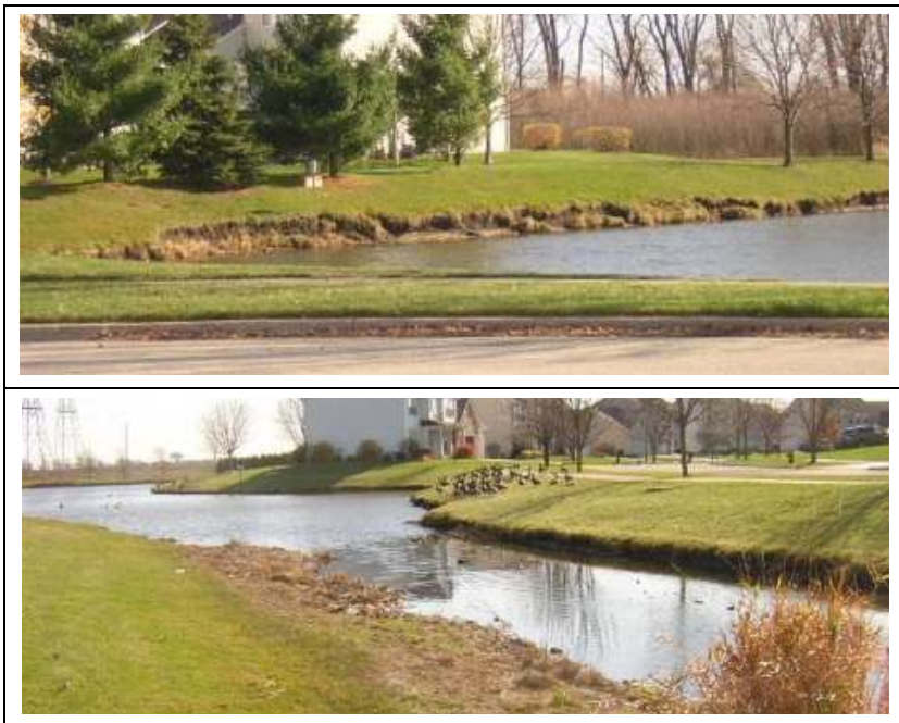
Figure 5-7. Sloughing and eroding shorelines at Oak Hill Pond, North Aurora. (Photos courtesy of Village of North Aurora)
