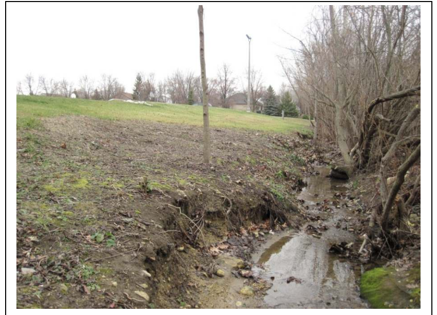
Figure 5-17. Upstream view of Hanks Creek bank conditions. Invasive brush has been cleared from the left but not yet from the right bank (December 2011).
