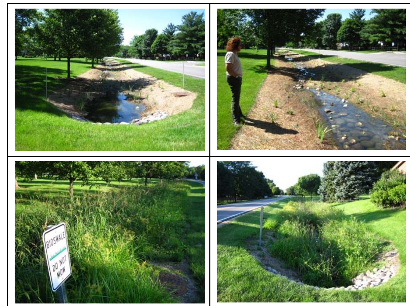
Figure 5-8. Previously installed bioswale along Hanks Road (top photos June 2011; bottom photos August 2011).
